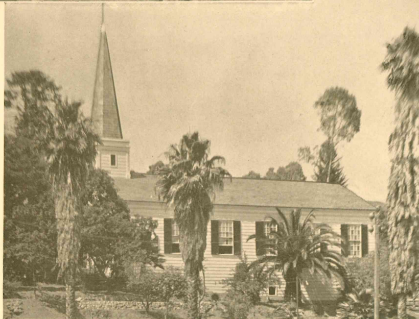
The Country Church as Seen from Hollywood Boulevard
